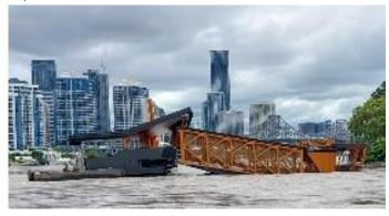
The walkway is supposed to swing downstream so debris won't hit it (see graphic below). It appears that feature didn't function properly on the new terminals which allowed debris to stack up against them.
